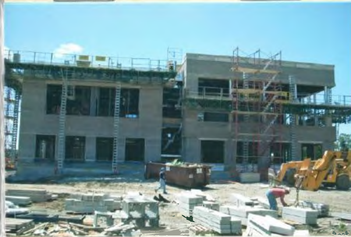
Constructing 4th Village Hall 2008-2009 2 Community Bldg 2 pics
