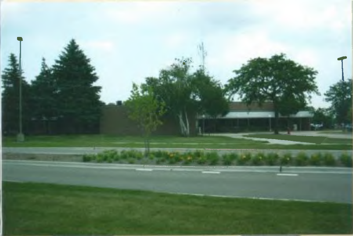
Old entrance To COUNThouse Old Village Hall #3 2009
