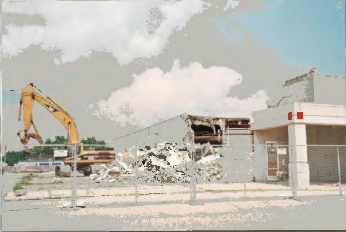
Demolition of K-mart Aug 2009 780 W Dundee
