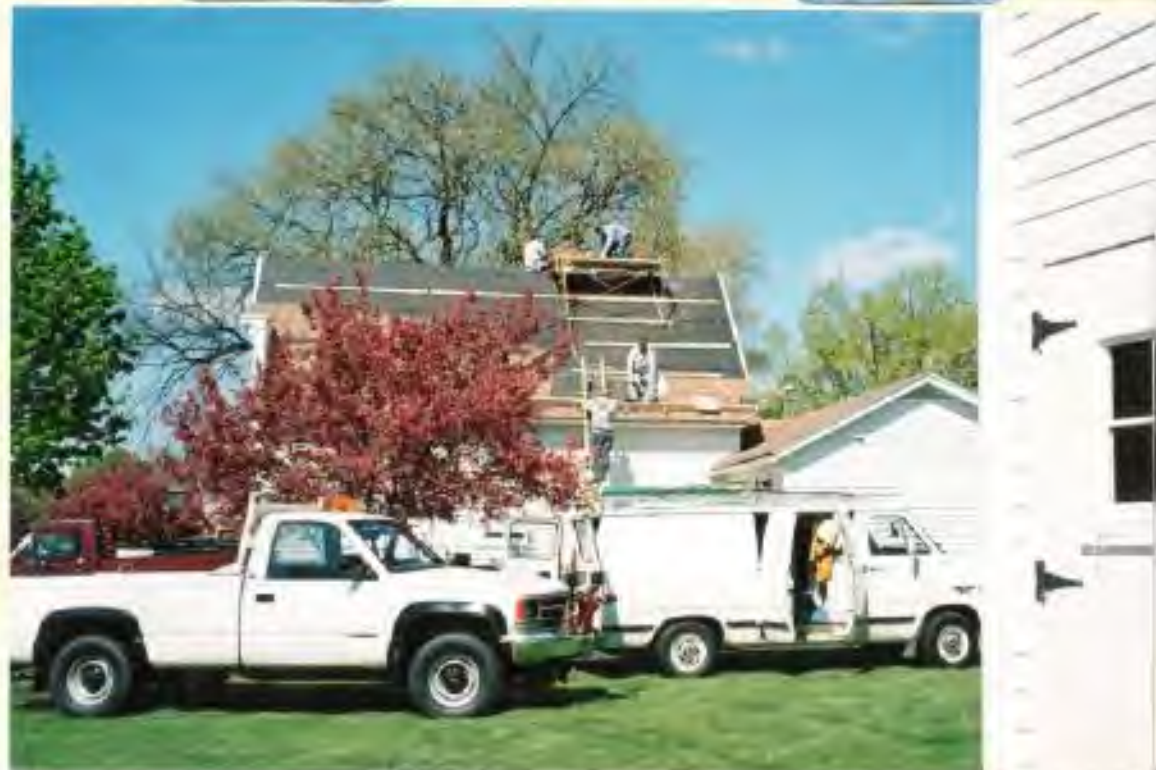
Reroofing Wheeling Museum Chamber Park
